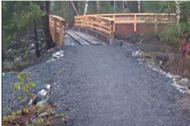
Figure 6-5—When installation is completed, the approach blends into the surrounding landscape.
