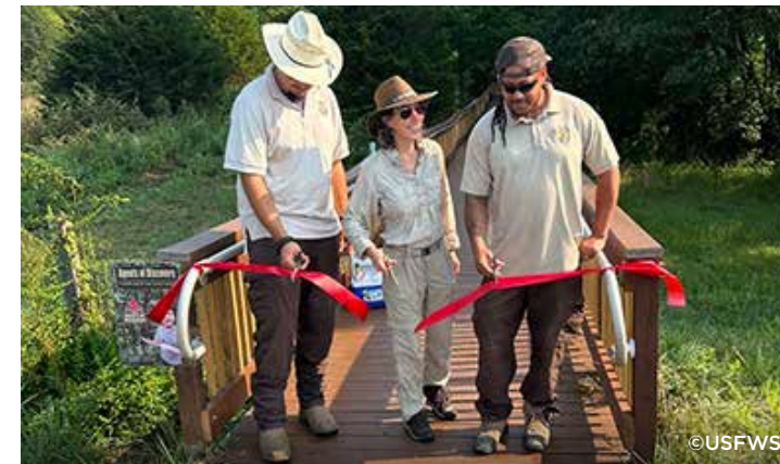
Project rehabilitated the Redington Boardwalk at Patuxent Research Refuge in Maryland after being closed for many years. Improvements to the boardwalk include new decking, handrails and benches.
